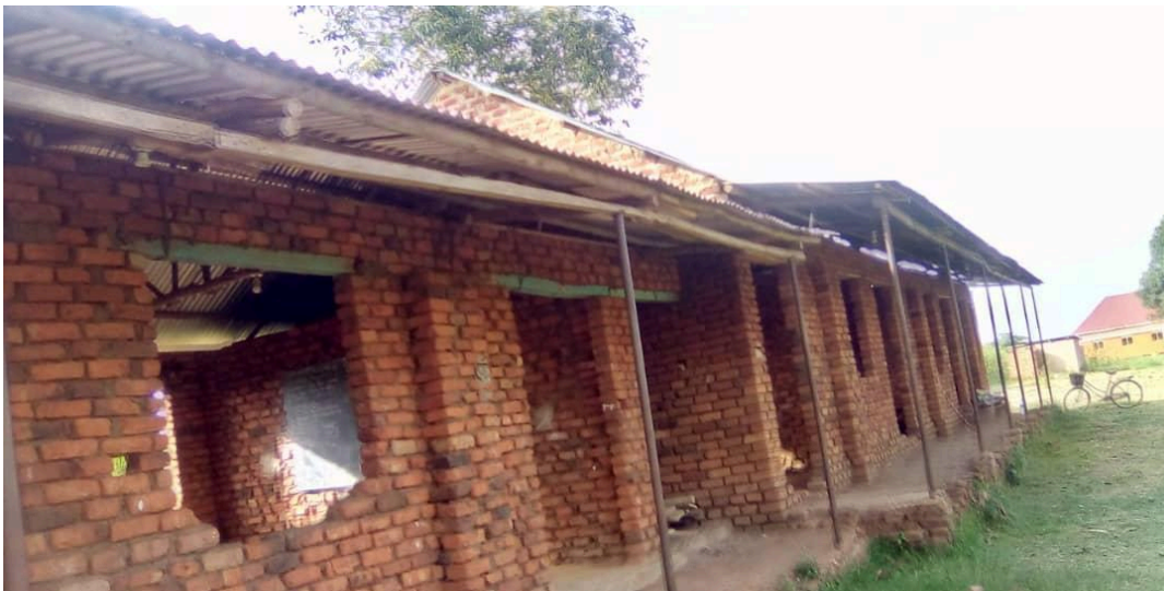
The school building at Glory FCIM Uganda
