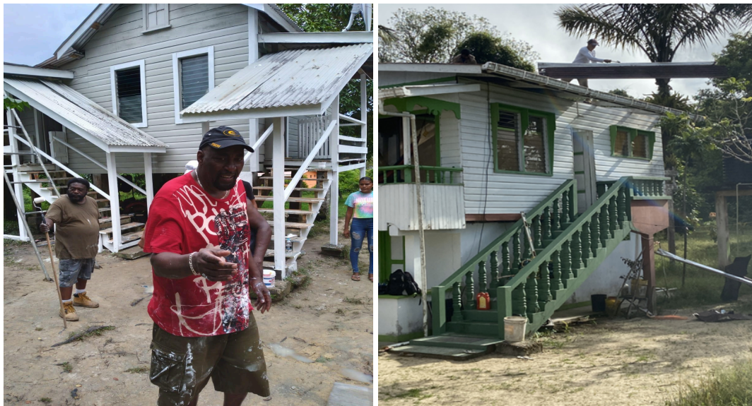
The mission team helping to rehabilitate homes in Guyana
